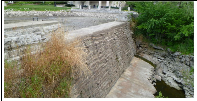
Existing Concrete Lined Channel at Railroad Crossing
