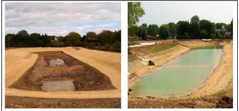
Wet Detention Pond Under Construction
