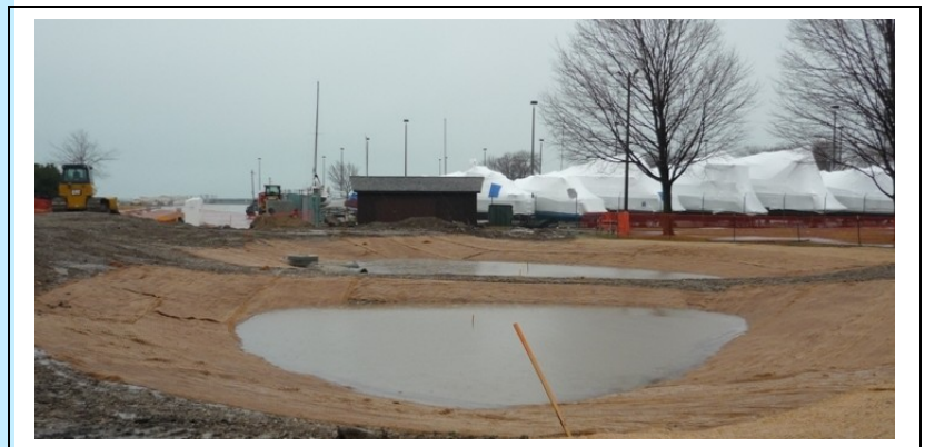
Raingarden/biofilter Device During-Construction and Rain Event
