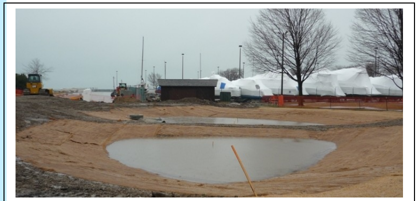
Raingarden/biofilter Device During-Construction and Rain Event
