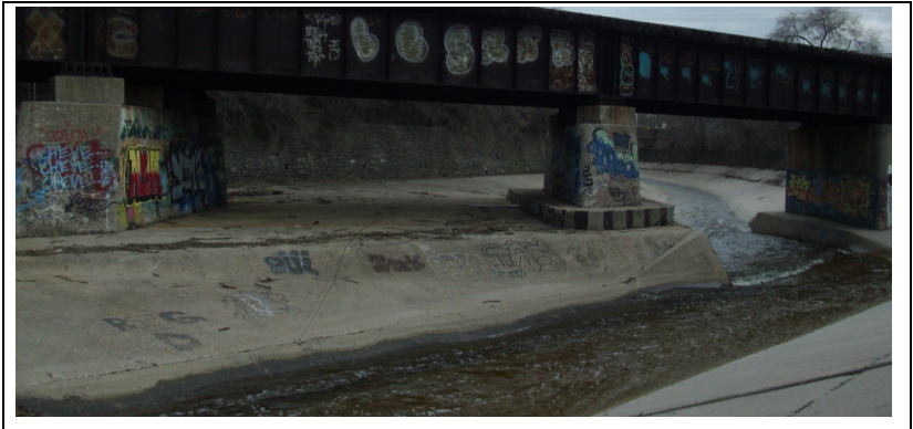
Existing Concrete Lined Channel at Railroad Crossing
