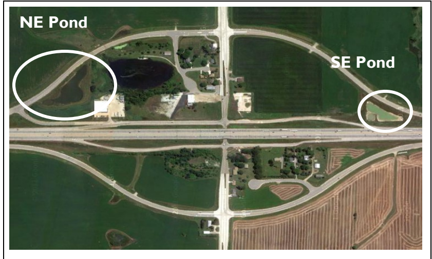
Aerial Photo of Ponds and Interchange
